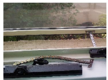
Chain winders replaced
