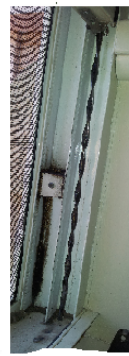
Spiral sash balances replaced
